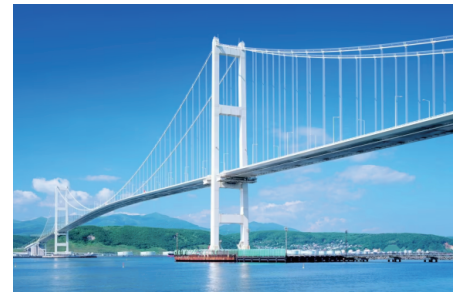
• 桥梁与大坝位移监测 Bridge & Dam Displacement Monitoring
